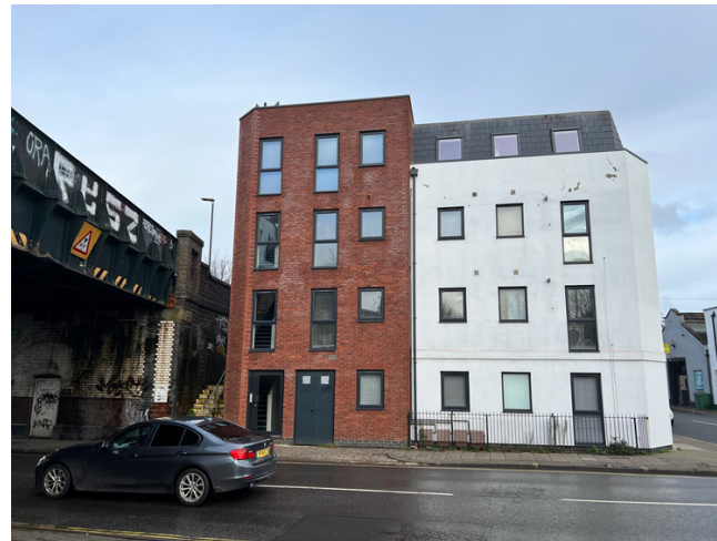
453 High Street (opposite the site)
