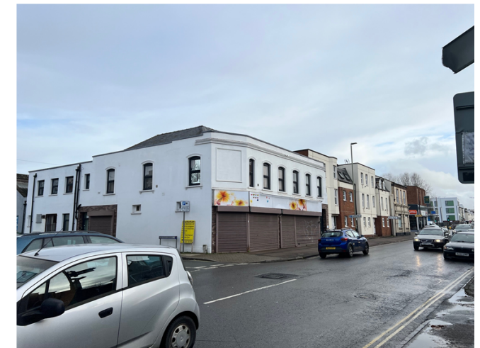
449 - 451 High Street (diagonally opposite the site to northeast)
